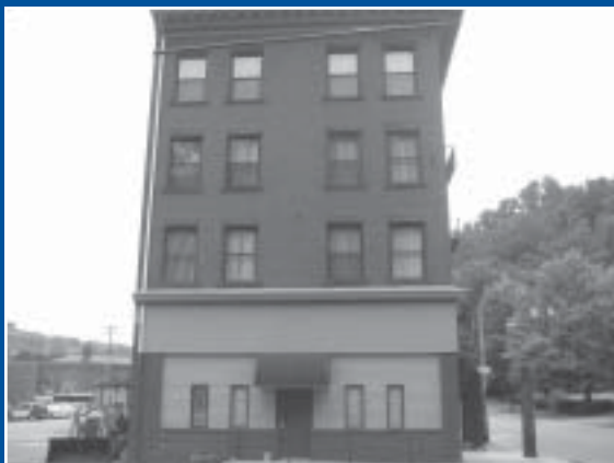
The old was made new with fresh paint, new awnings, pointing, modern lighting and ramps
